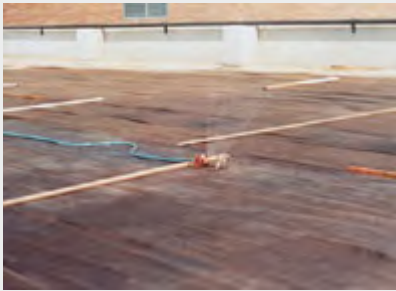
Figure #1. Covering wet burlaps & water sprinkling
