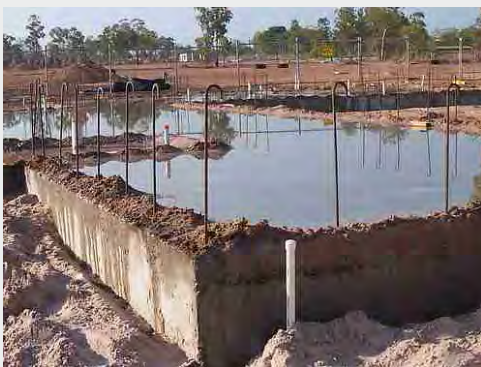
Figure #2. Ponding or immersion & sand curing
