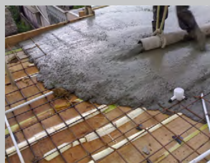
Figure #4. Reduced manpower needed for consolidating and placing concrete.
