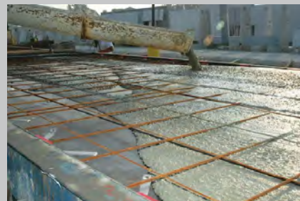
Figure #2. Placing concrete using truck chute which is concrete flowing freely on the slab.
