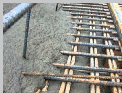
Figure #3. Congested reinforcement concrete completely filling and achieving full compaction.
