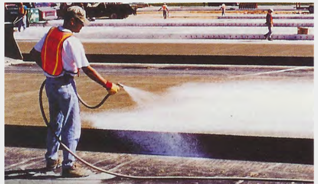
Figure #4. Liquid applied evaporation reducers
