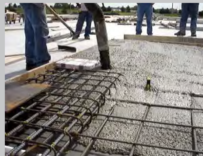
Figure #1. Placing concrete using pump without any using mechanical vibration.
