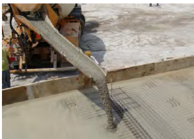
Figure #1. Truck Mixer Chute
