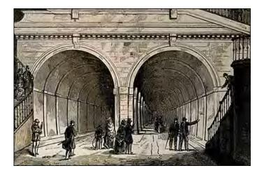
Brunel carefully placed several tons of his cement into the river when the tunnel roof collapsed. This sealed the break and Brunel was able to pump the brick-built tunnel dry and then reline parts of it with mortar made with Portland cement. Despite the problems with its construction, this was the world's first significant underwater tunnel.
